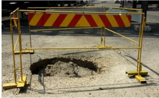
Good practice: Inter-linking steel frames
